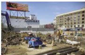
Construction of The Crossings - Bronx, NY
